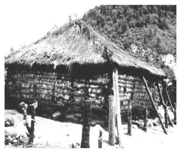
Fig. 1: Wattle and daub structure, after a heavy earthquake in Guatemala (Minke 2000)
